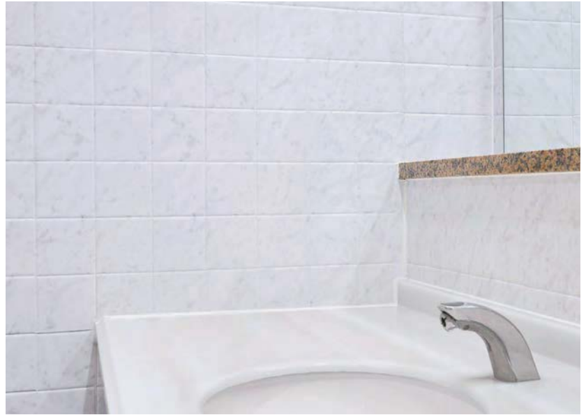
Restroom refurbishment / ST-024TIL
